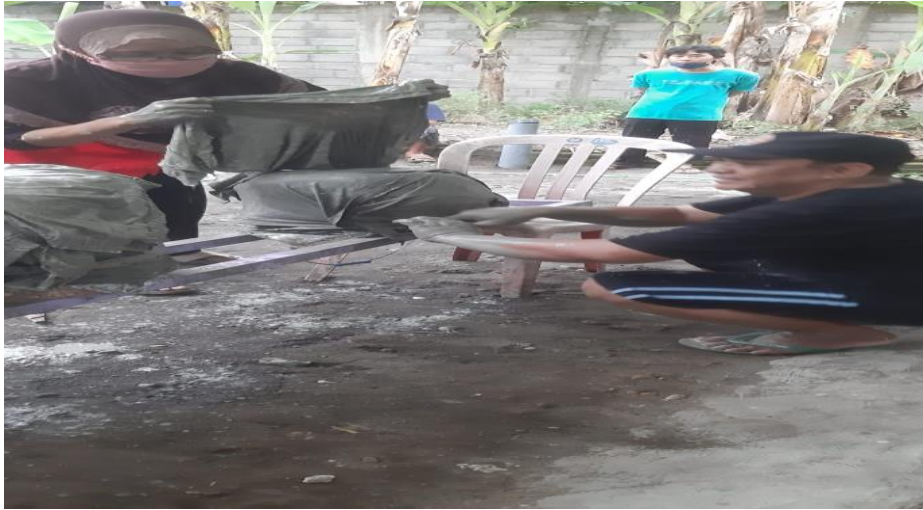
Figure 6. Placing the cemented fabric in the mold
