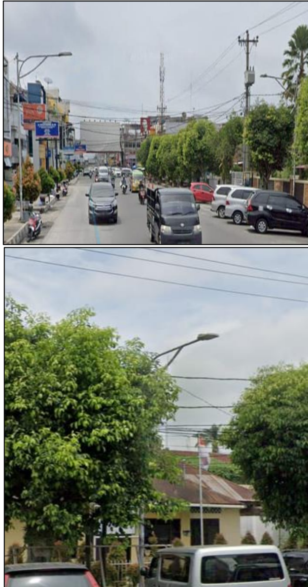
Figure 8. Condition of PJU covered by trees
